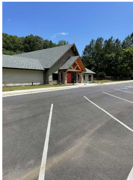
Church abutting south property line
