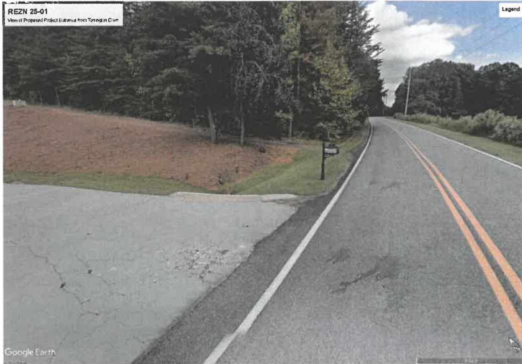
View of Project Entrance from Torrington Drive
