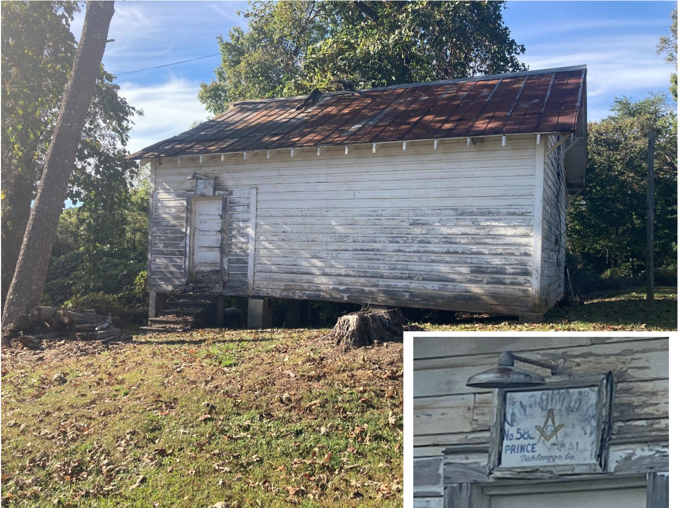
Figure 1-5 - 245 Goudlock Street, unknown construction date for GNAHRGIS ID #281040 – Former One Room School house and Gold City Masonic Lodge.
