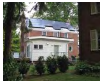
Solar panels have been installed at the rear; however, because the house is situated on a corner, they are highly visible and negatively impact the historic character of the area.
