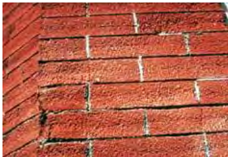
Sandblasting brick or stone surfaces using dry or wet grit or other abrasives. These methods of cleaning permanently erode the surface of the material and accelerate deterioration.
