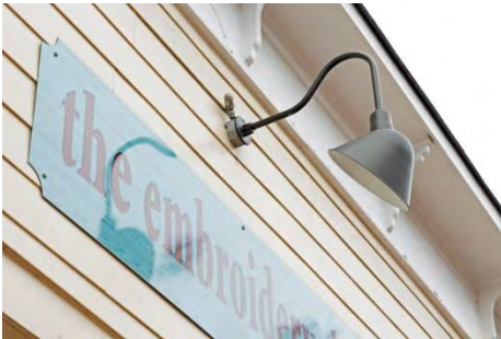
Example of goose neck exterior lighting that is appropriate.
