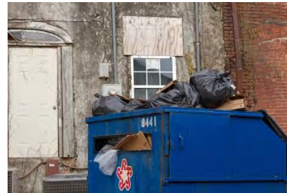
Example of unscreened service area.
