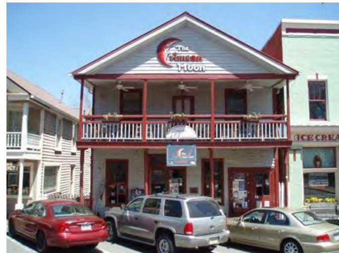
Figure 6. John A. Parker Storehouse, 1858.
