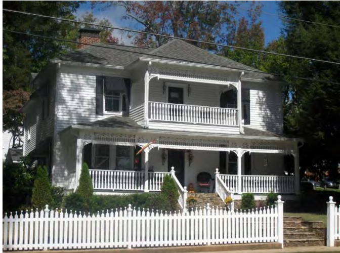
Figure 16. Residential structure in the Historic District.
