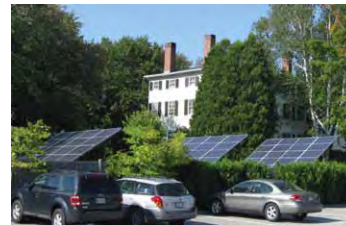
Although solar panels are installed behind a parking lot, the panels negatively impact the historic property.
