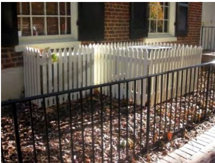
Example of appropriately screened HVAC units.
