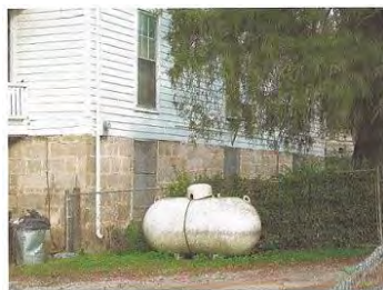
Example of inappropriately screened external utility gas tank
