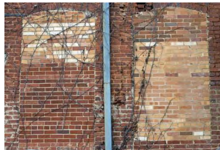
Brick infill does not match original in texture, color or pattern.
