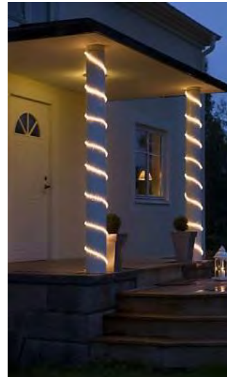
Rope lights are not appropriate on historic exteriors.
